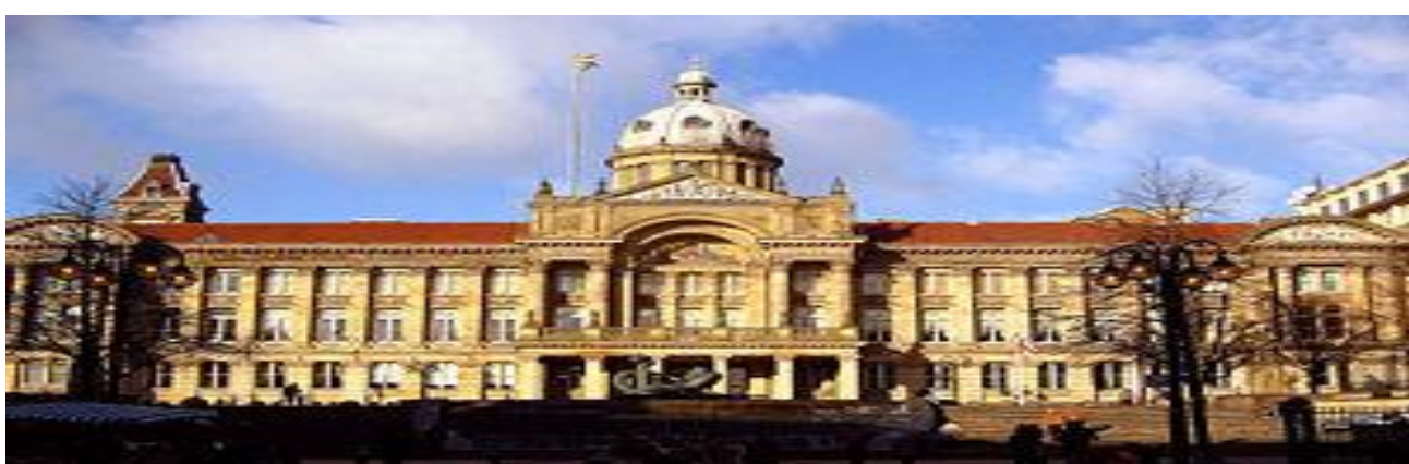
Councils in England are in buildings such as the Birmingham Town Hall.
