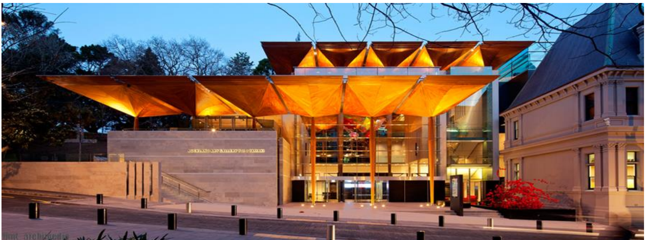
The modern section of the Auckland Art Gallery, completed in 2011
