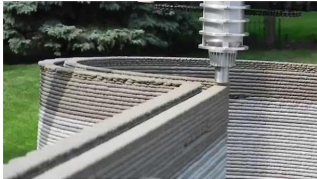
*Figure 2. An example of how concrete should be laid in even layers without spreading*
